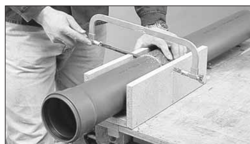
(Diagramme 19) Cutting to length with a fine-toothed saw
