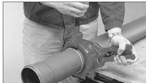
(Diagramme 18) Cutting to length with a cutting and chamfering tool
